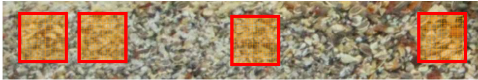
Figure 3. Measurement zone along pile top surface
